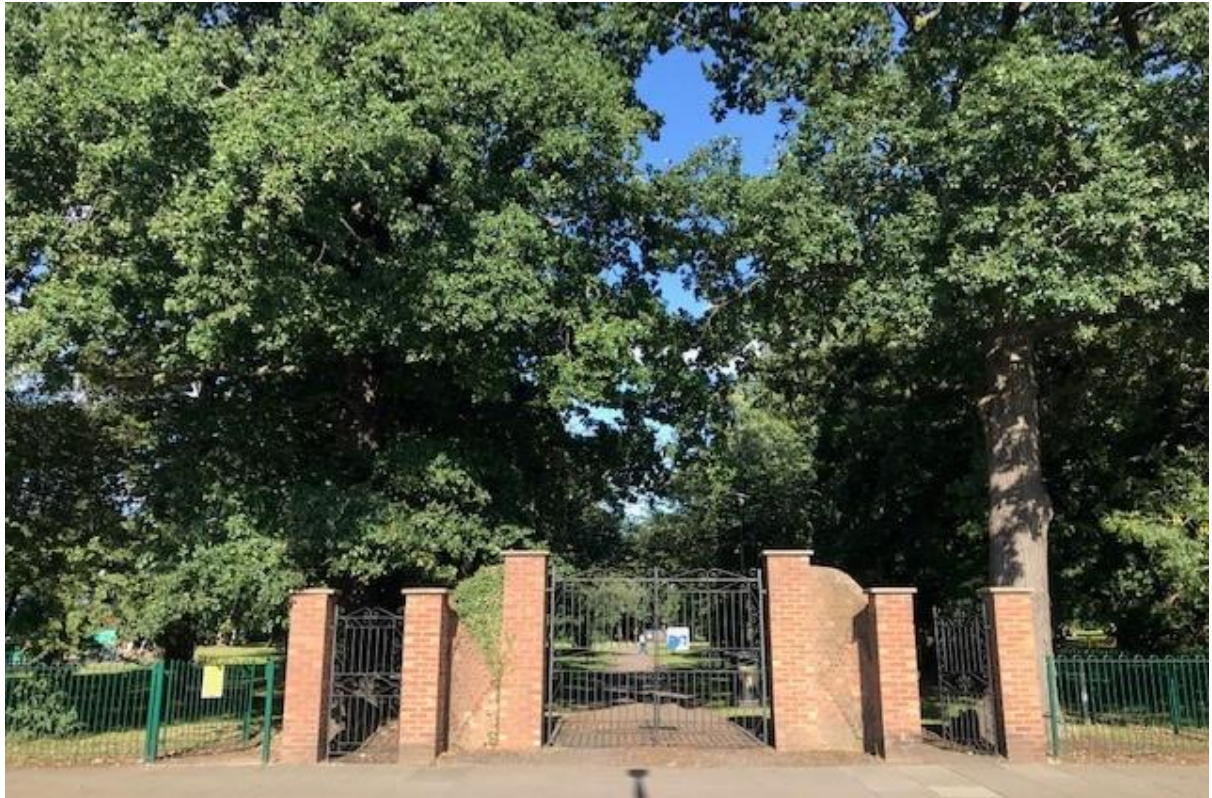
Main entrance gates to Dilkes Park c2020 Image Heather Hunter
